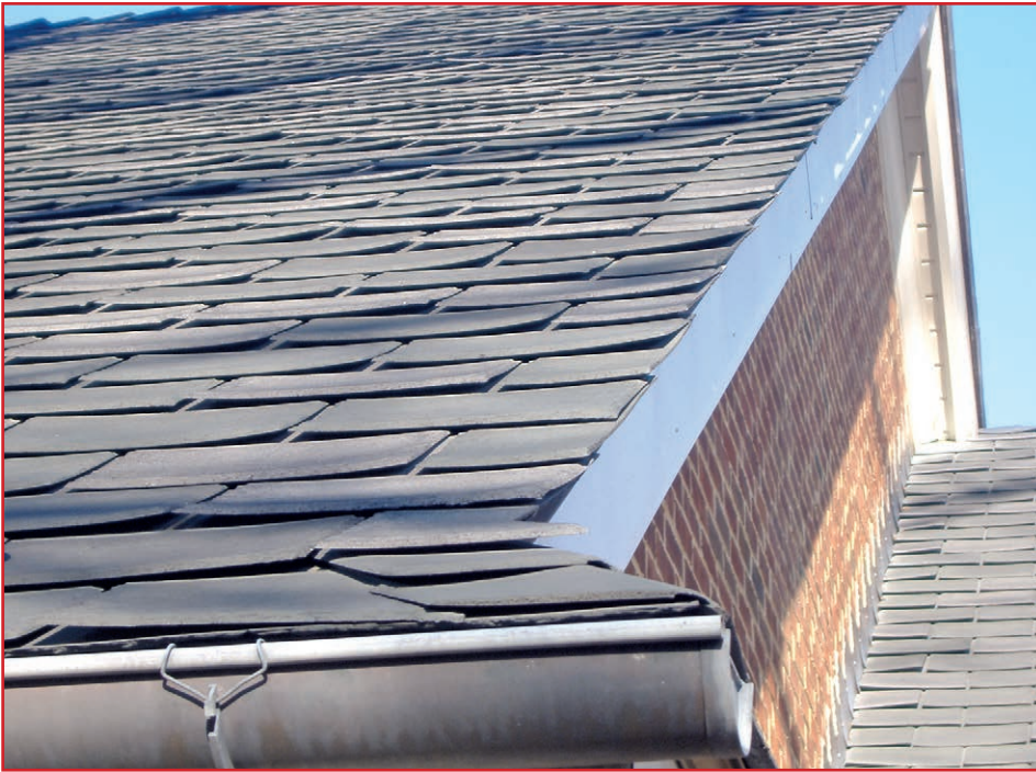
Figure 4 – Warped polymer shingles detract from a roof’s appearance and impact its watertightness. Photo courtesy of Alan Buohl, GSM Roofing, Ephrata, PA.
