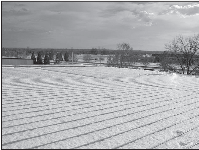
Figure 3 - Submerged SSMR after hailstorm.
